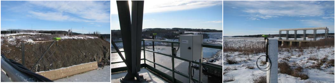
Left: A GS100 antenna mounted on the face of the Diversion. Centre: A GS100 located on the Main Intake. Right: GS100 located in a stable area with good satellite visibility.
